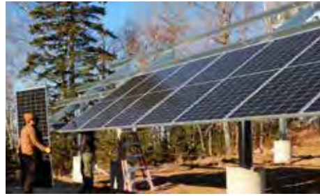
Installing the new solar array.
